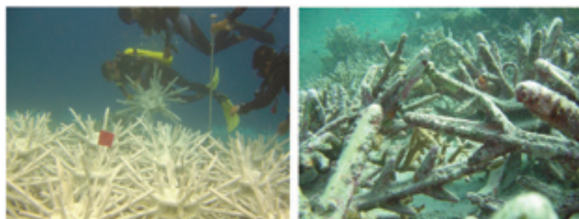
Fig. 2.2 – Eco reef modules being placed on a damaged reef and 2 years after deployment (image © eco reef.com).
