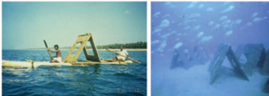
Fig. 1.4.9. – Ferroconcrete artisanal fishery reef units, Kerala, southern India (Source: left: Alternative Technology; right: Antony Jensen, NOC).
